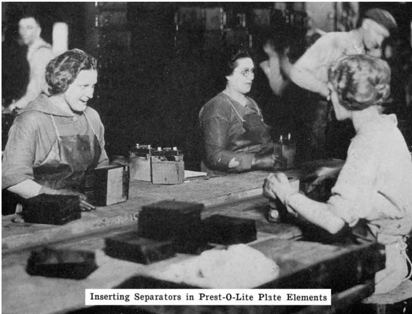
**Inserting Separators in Prest-O-Lite Plate Elements**
