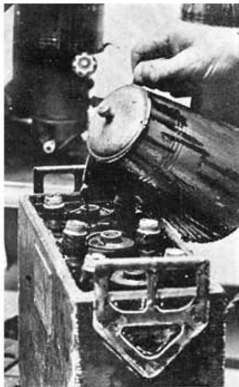
Fig. 229. Pouring Compound on Lower Covers
