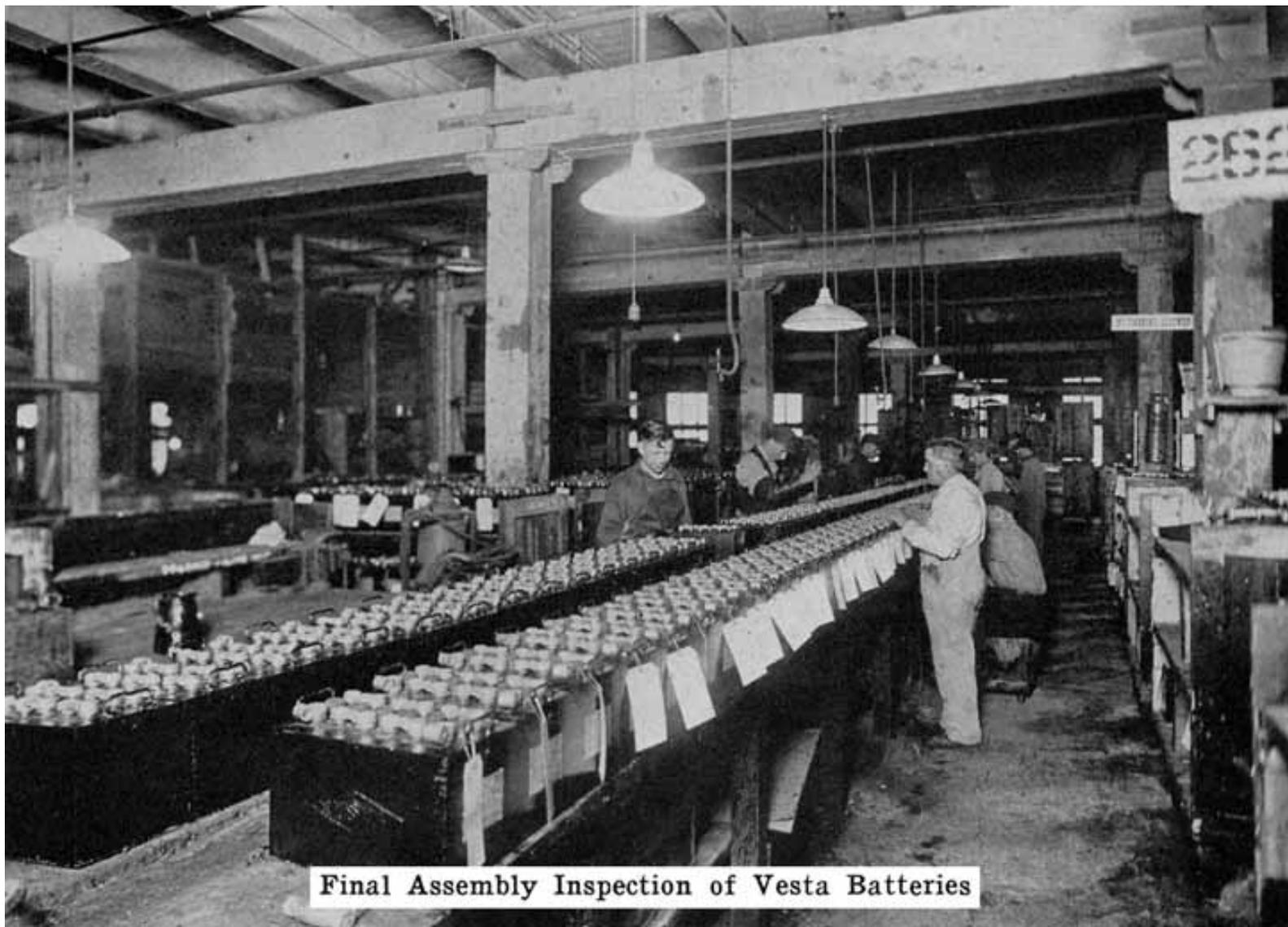
**Final Assembly Inspection of Vesta Batteries**
